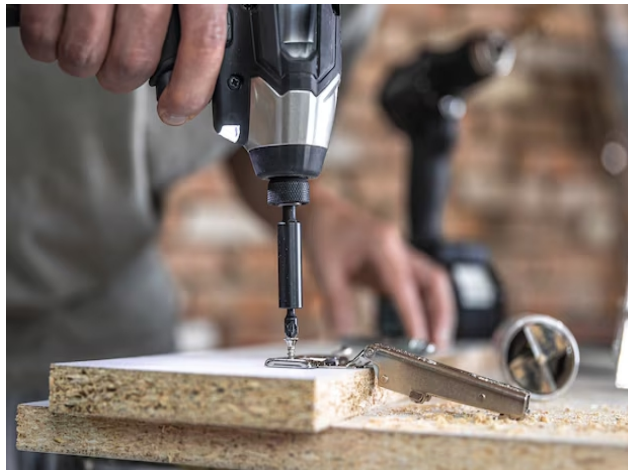
Fig. 2.35: Drilling and Fastening
