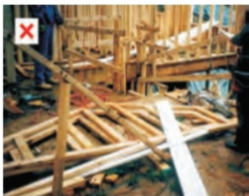
Fig. 7.35: Do not stack the waste material at a place; dispose it regularly
